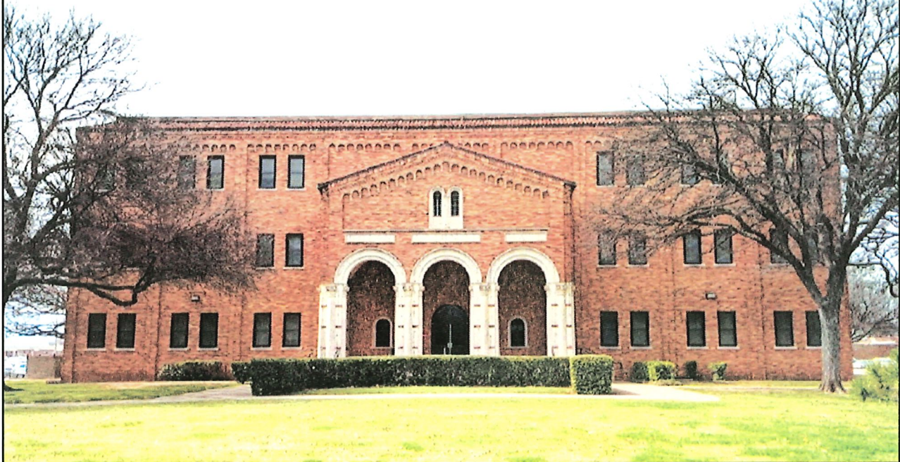
Bolin Hall – East Elevation
