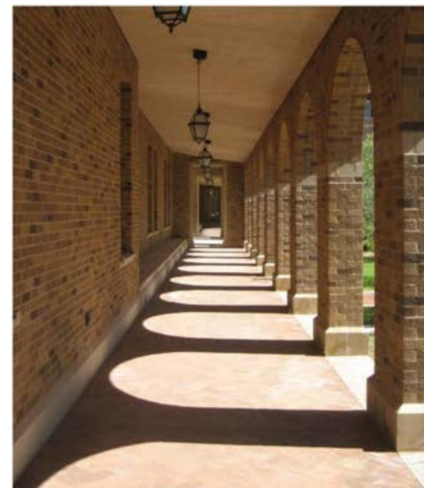
Above: Experimental Sciences (completed 2006) is a more recent example of the implementation of colonnaded arcades onto campus facilities. Here, a canted plaster ceiling is in place over the arcade.
