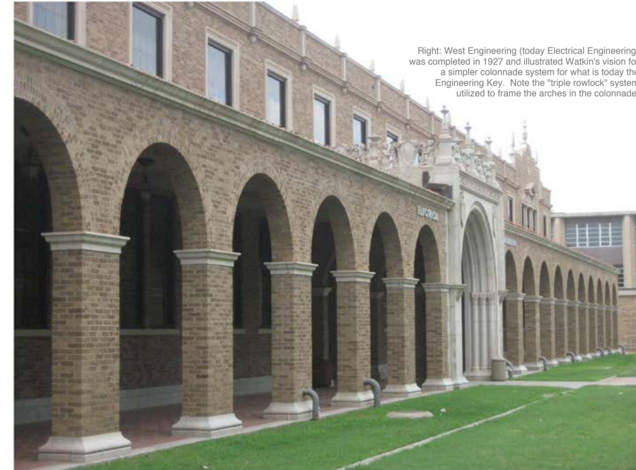
Right: West Engineering (today Electrical Engineering) was completed in 1927 and illustrated Watkin's vision for a simpler colonnade system for what is today the Engineering Key. Note the "triple rowlock" system utilized to frame the arches in the colonnade.
