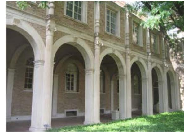
Above: The south colonnade to the Administration Building (1925) is an example of the use of engaged columns in the colonnade itself, as well as domical vaulting over the arcade itself.
