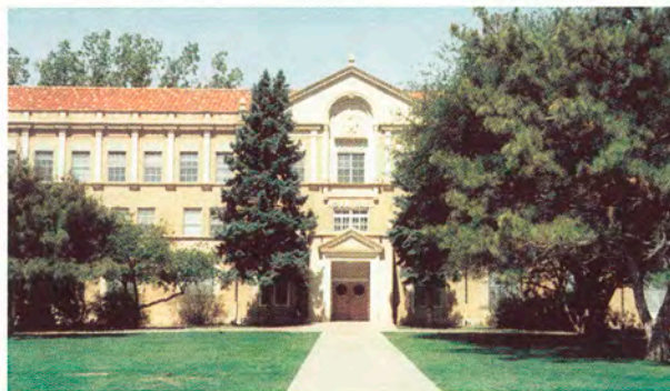
Gable at Entry
