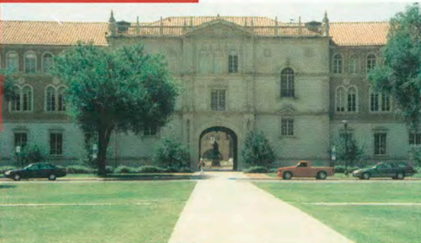
Limestone Base and Entry
