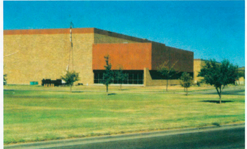
Central Heating and Cooling Plant I
