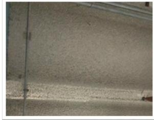
Insulation (beige) (fireproofing) on pan deck in basement and Floors 1-9
