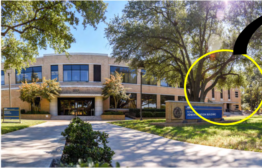
Sol Mayer Administration Building
