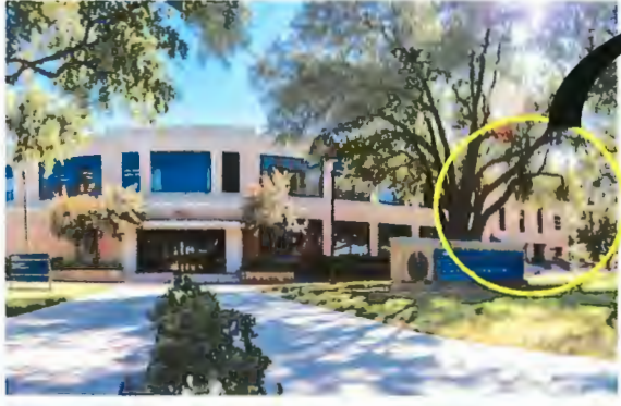
Sol Mayer Administration Building
