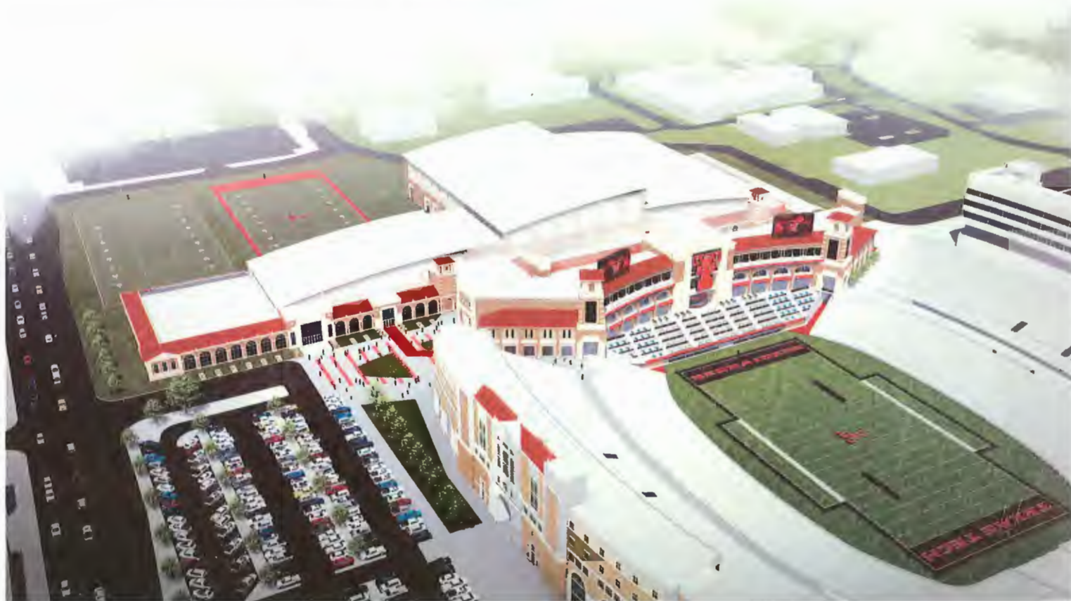
Aerial 05-05-2022 Womble Football Center and South End Zone
