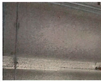
Insulation (beige) (fireproofing) on pan deck in basement and Floors 1-9
