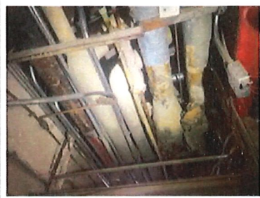
Domestic water line fitting (gray, hard) in Basement and pipe chases between floors
