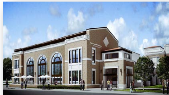
Rendering View of the Dining Facility (Exterior)
