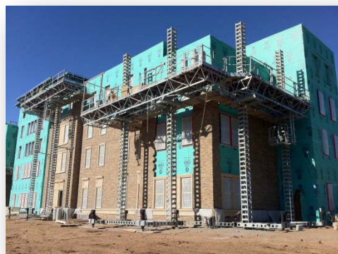
View from the Southwest
